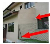
Movement cracks observed at wall joint between extension and original rear wall.
